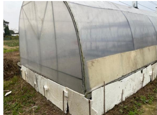
Figure 9 Polystyrene pasted for thermal insulation
