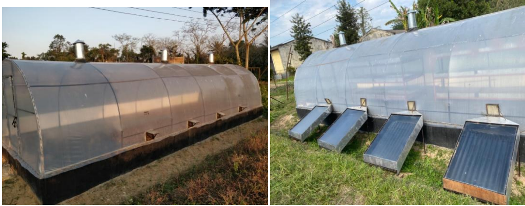
Figure 12 Air inlets fitted with flat bed collector
