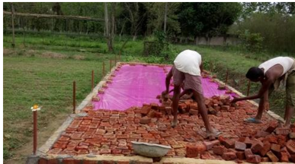
Figure 7 LDPE sheet layering work in cement concrete base construction
