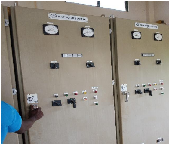
Motor starting panel
