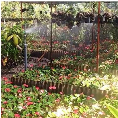
Figure 6 Automatically controlled sprinklers installed at parental plant station
