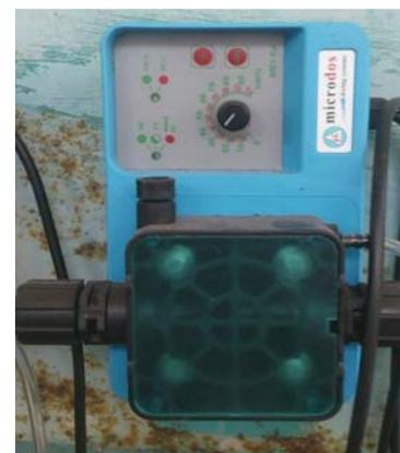
Figure 12 Automatic device to install the percentage of chlorine in drainage water of the abluion
