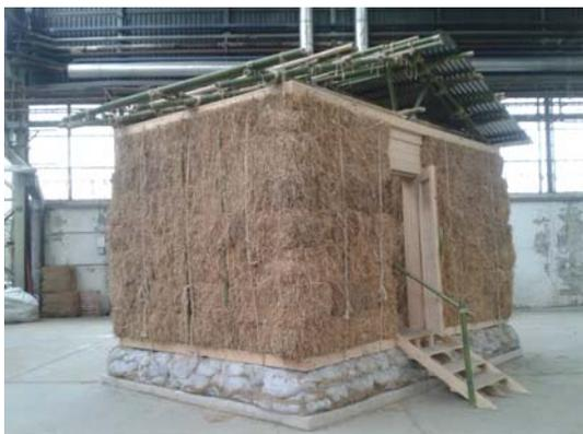
Figure 12 Housing module with bearing straw bales, realized with the Anpilpay 2.0 press
