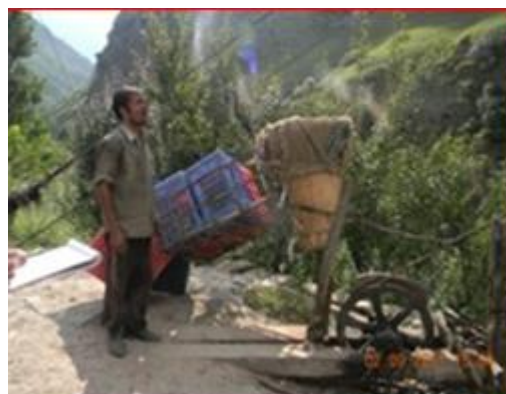
Figure 5 Rope ways used for material handling
