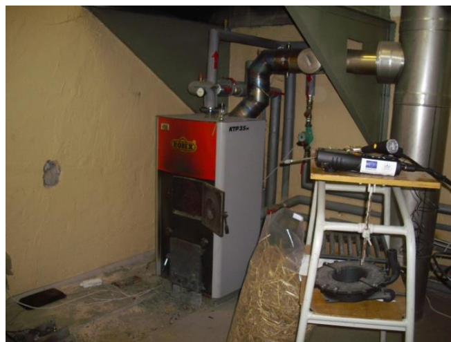
Figure 3 Hot water boiler KTP 256 m (ROJEK manufacturer)
