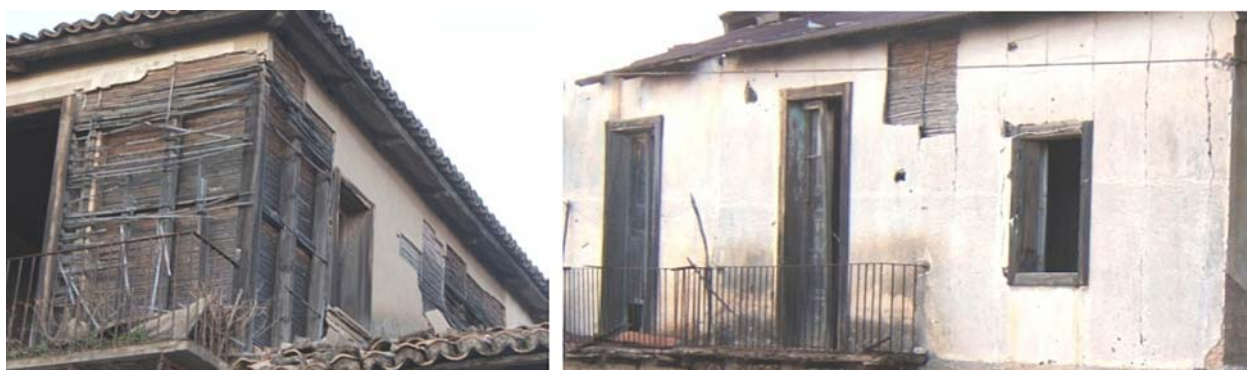
Figure 2 Rural buildings in the south of Italy with external walls panelled with Arundo donax L.
