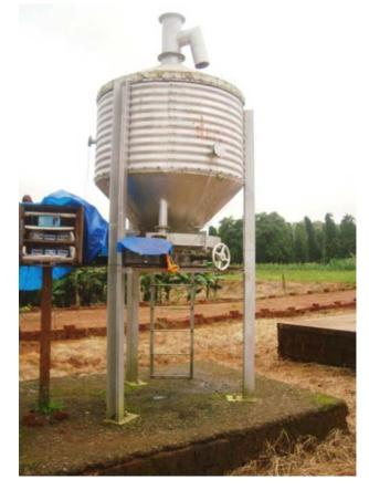
Figure 1 Galvanized iron corrugated structure for storage of wheat
