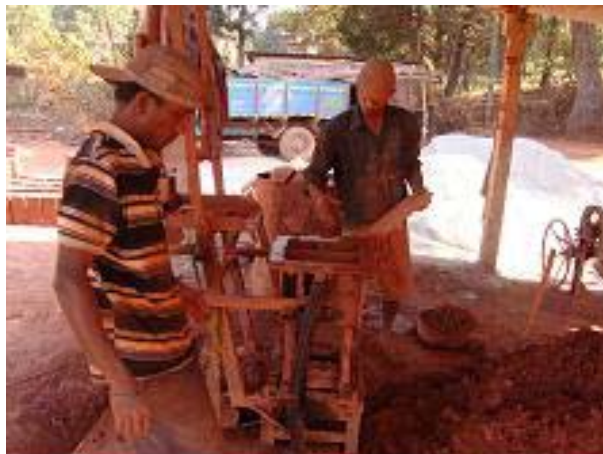
Figure 2 Laterite stone scrap block making machine while in operation
