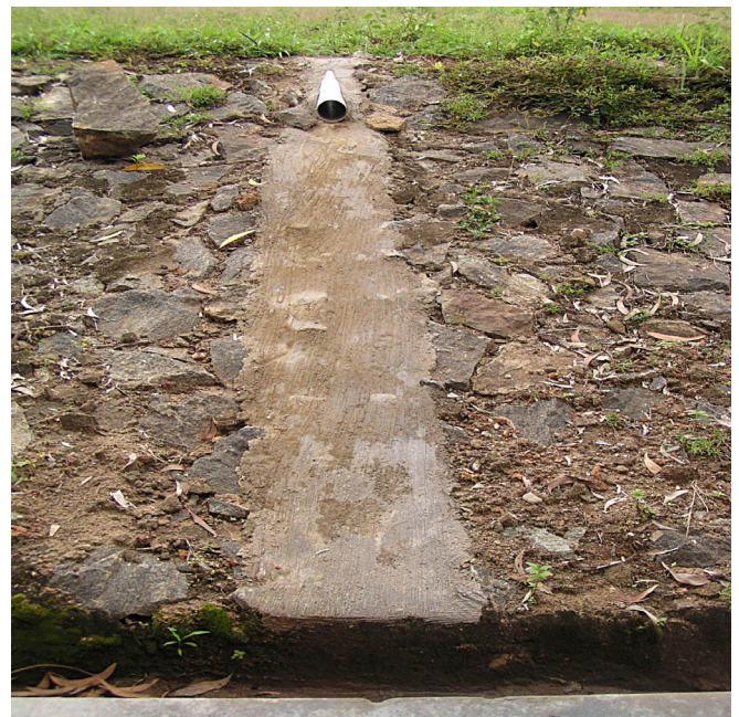
Figure 1 Cement plastering at the stone pitched area
