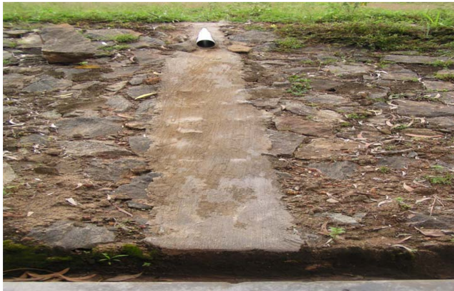
Figure 1. Cement plastering at the stone pitched area
