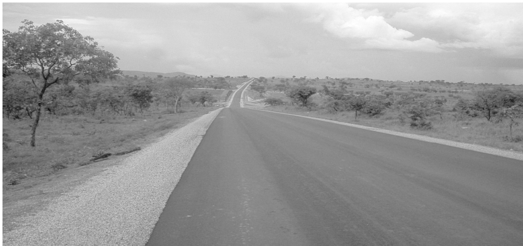
Picture 1 View of road after construction
