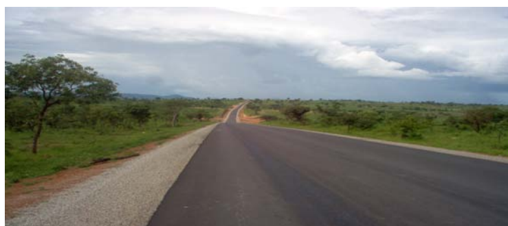
Picture 1. The view of road after construction
