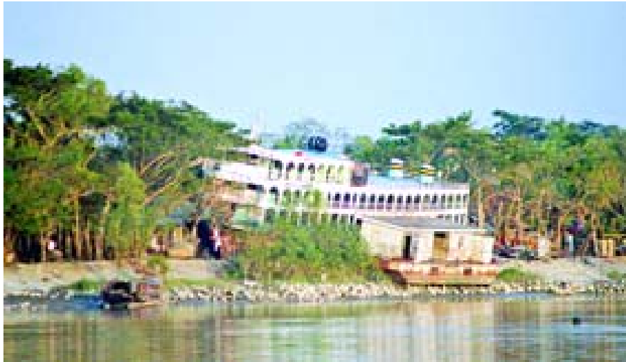
Fig.3. Three story ferry comes on the ground due to storm surge of Sidr 2007 (Nayadigonta)
