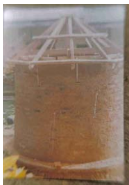
Figure 5: Completed roof truss of the silo
