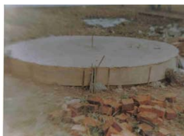
Figure 3 Round concrete floor on stone foundation
