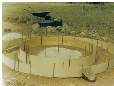
Figure 2: Veneers and iron rods used to mark the circular foundation
