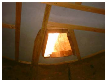
Figure 6: Loading chute attached to the roof truss
