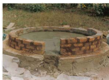
Figure 4: Setting of bricks in progress
