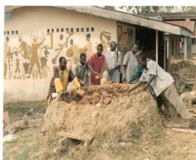
Figure 1: Dried termite mound bricks being set for burning in a mud-kiln
