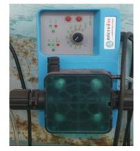
Figure 12 Automatic device to install the percentage of chlorine in drainage water of the ablution
